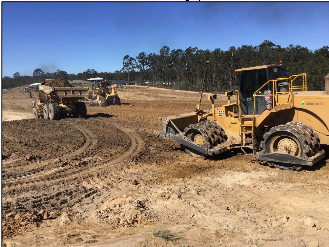
Picture 2: View of Filling Operations
