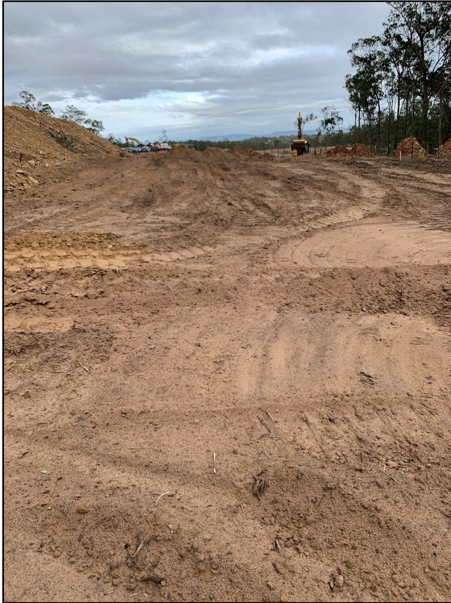
Picture 1: View of Stripping Operations
